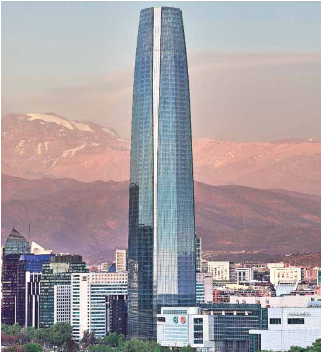
Costanera Center, Santiago, Chile
